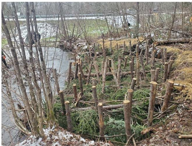
**Figure 10: Bank stabilization works on the Coxs Brook, November 9th, 2023 (Photograph D. LeBlanc)**
