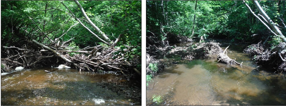
Figure 70: Before and after photos of debris jam below the fish ladder.
