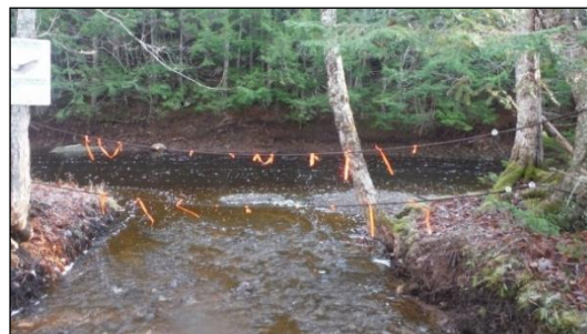
Figure 104: ATV access blocked, Scoudouc River.
