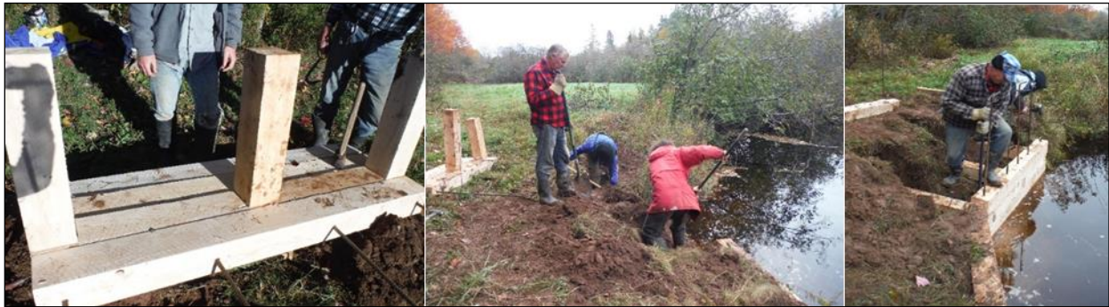
Figure 100: Retaining wall construction in 2015, Scoudouc River.
