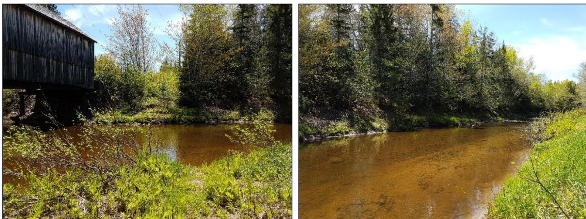
Figure 17: Site photos of water quality monitoring station ShdE, spring 2018.
