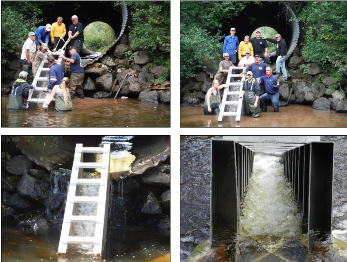
Figure 68: Installation of the fish ladder in 2015 on the McQuade Brook.
