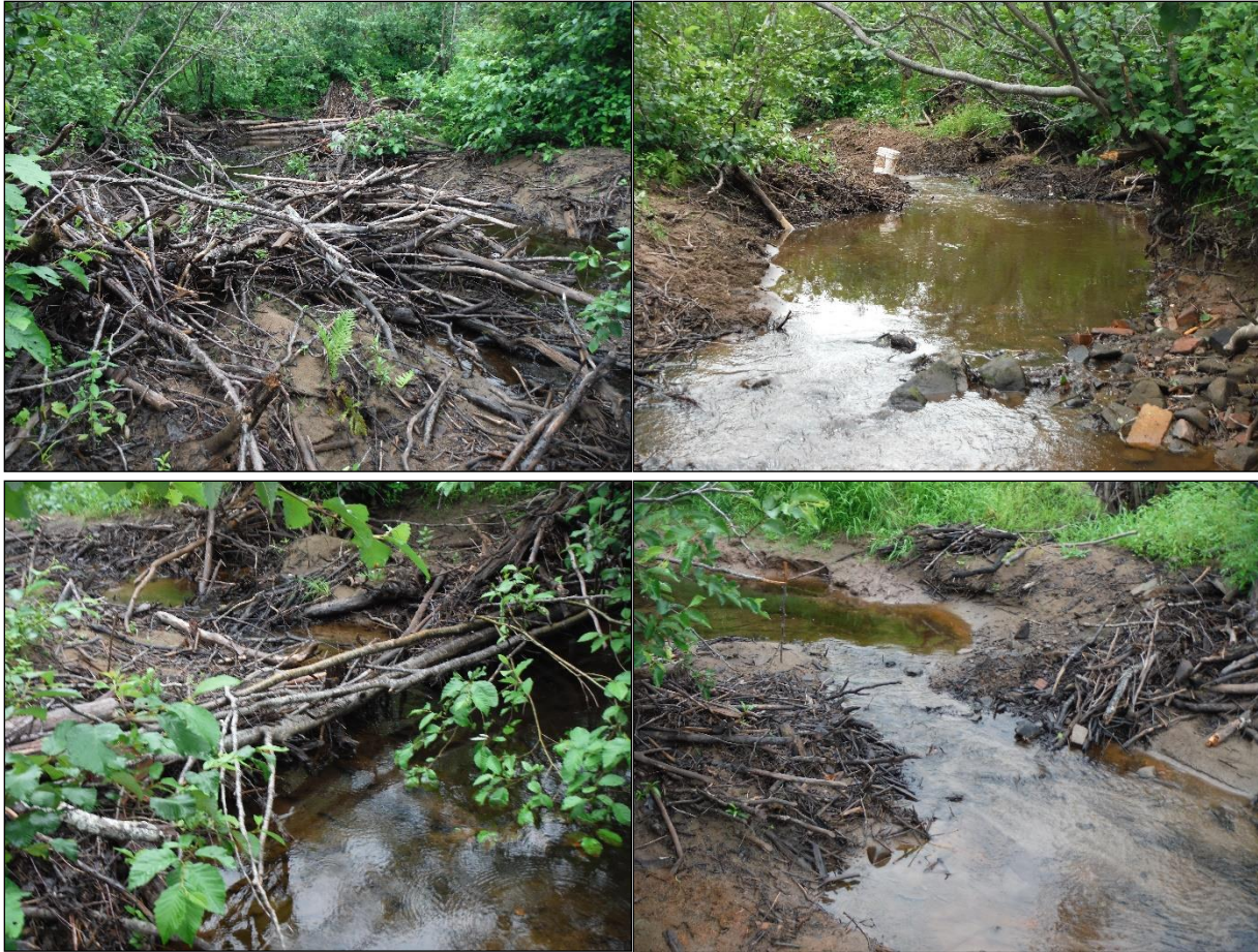
Figure 69: Before and after pictures of debris jam in the McQuade Brook, 2014.
