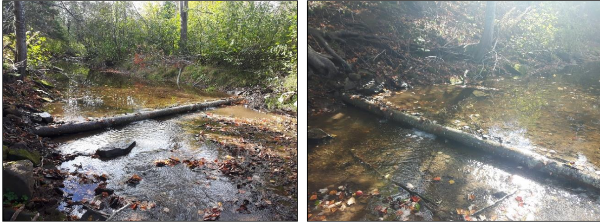
Figure 72: Digger logs installed in the McQuade Brook, 2016.
