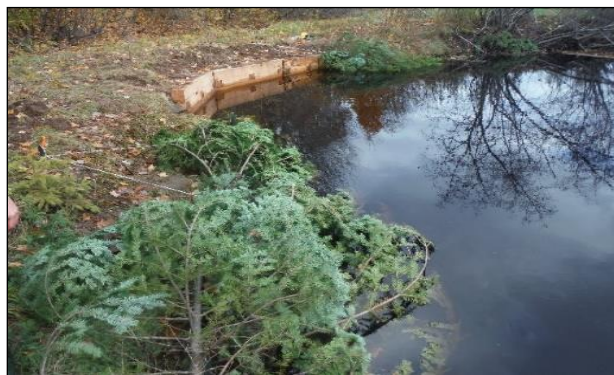
Figure 101: Retaining Wall Scoudouc River.
