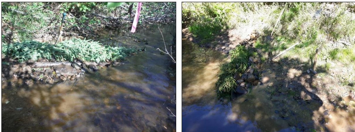
Figure 71: Deflectors installed in the McQuade Brook, 2016.
