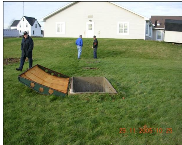
Figure 98: New septic system at Arsene Richard Seniors Home, Scoudouc.
