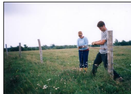
Figure 30: Cattle fence work.
