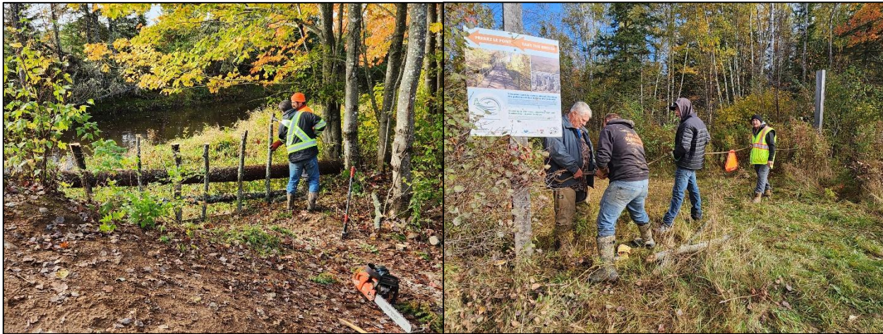
Figure 35: Volunteers from the Kent ATV Club help with the installation of logs and cables.
