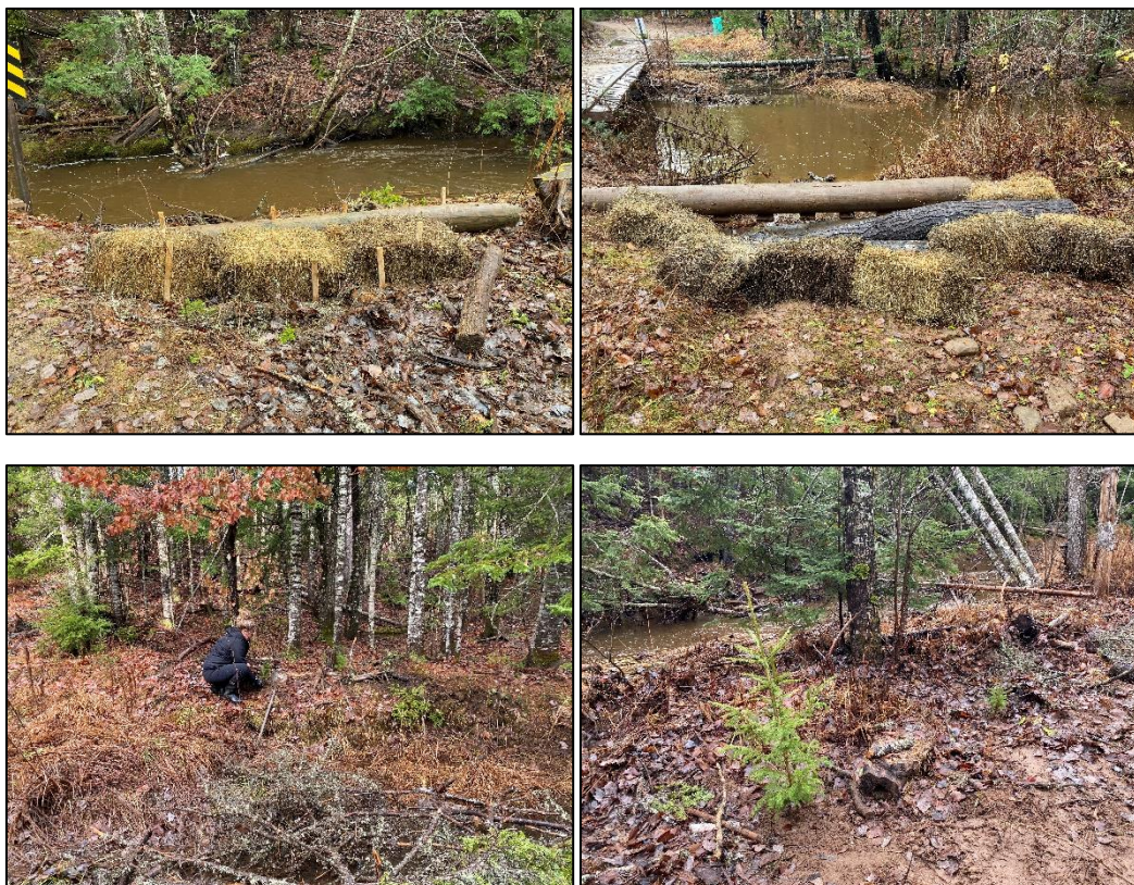
Figure 51: Large logs and hay bales were used to block access to the Calhoun Brook (top). Trees were also planted on site (bottom).
