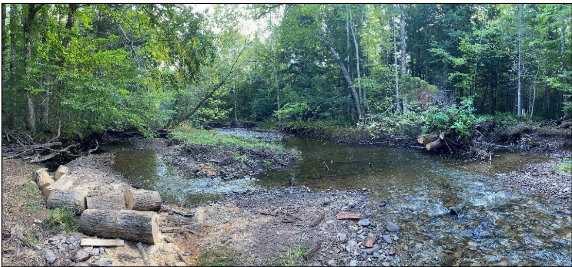
Figure 37: Debris jam after removal.
