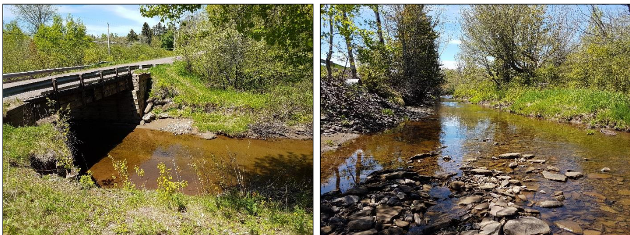
Figure 16: Site Photos of the Water Quality Monitoring Station ShdC, spring 2018
