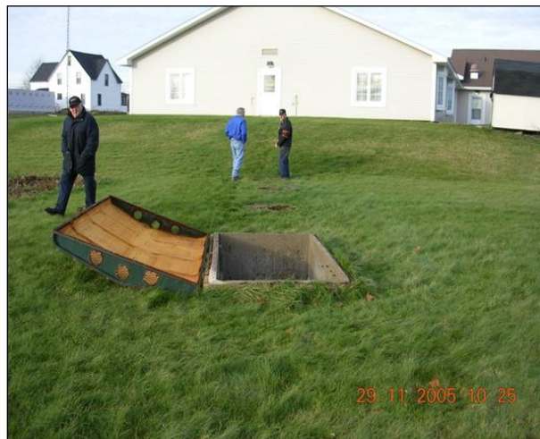
Figure 108: New septic system at Arsene Richard Seniors Home, Scoudouc
