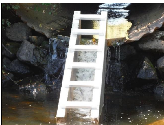
Figure 72: Installation of the fish ladder in 2015.
