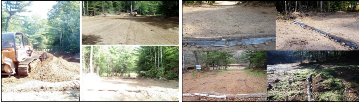
Figure 113: Restoration work done on ATV trail at Edna's pond, 2017
