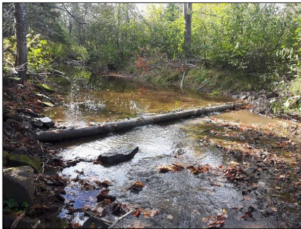
Figure 80: Digger logs installed in the McQuade Brook, 2016
