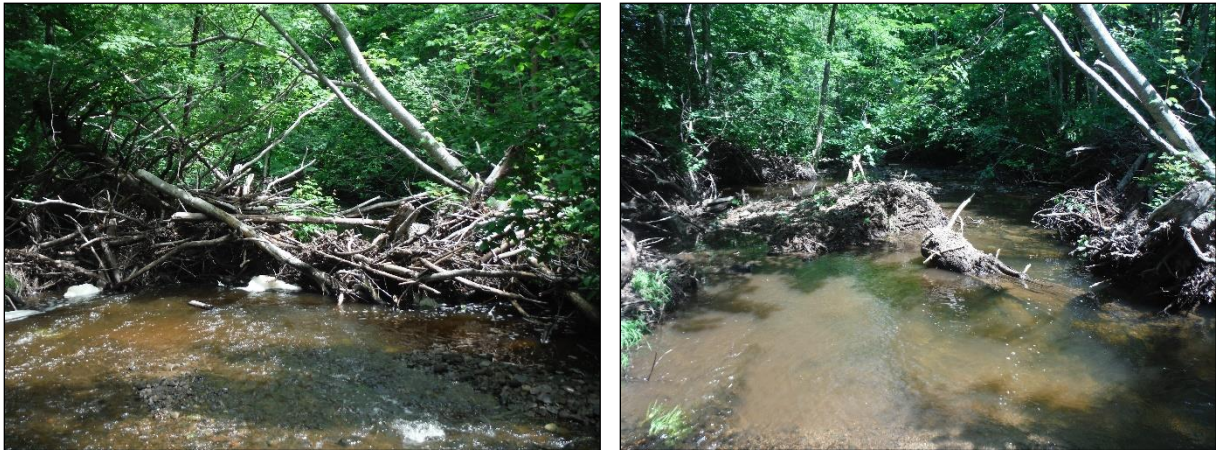
Figure 78: Before and after photos of debris jam below the fish ladder
