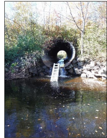
Figure 71: Fish ladder on the McQuade Brook
