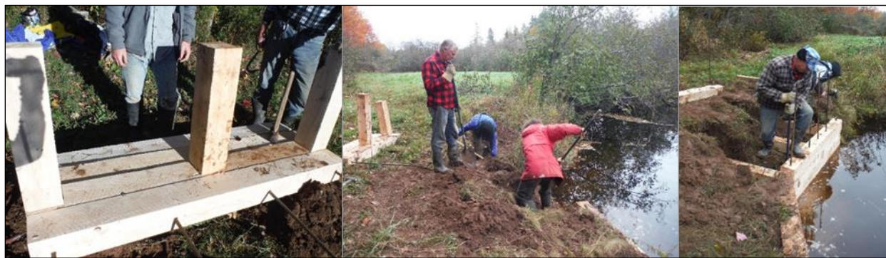
Figure 110: Retaining wall construction in 2015, Scoudouc River
