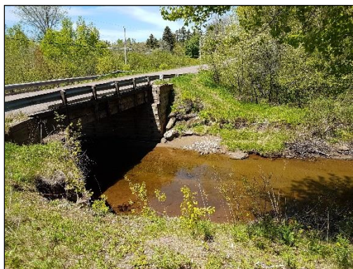
Figure 22: Photo of the Shediac River in the Cape Breton area, survey performed downstream of bridge
